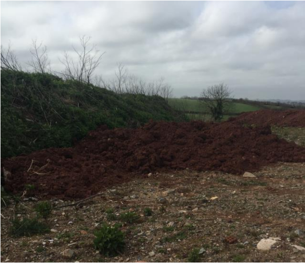
New top soil that that been brought onto the site – this is in the centre of the site, outside of the Temporary Soil Storage Area
